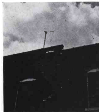
TRANSMISSION LINE FROM RCA VICTOR "TERRA-WAVE" POLICE RADIO TRANSMITTER TO THE ANTENNA AT SPRINGFIELD, MO.
