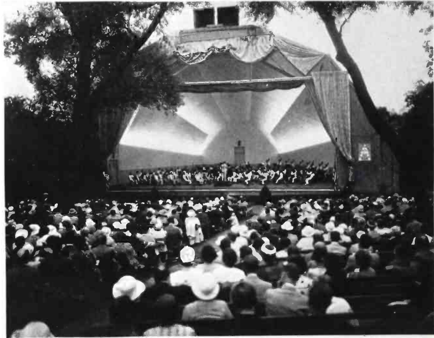
A CONCERT IN PROGRESS AT ROBIN HOOD DELL, PHILADELPHIA. THE TWO DIRECTIVE BAFFLE RCA VICTOR LOUDSPEAKERS ATOP THE SHELL SERVE THE REAR PORTIONS OF THE AUDIENCE, AND ARE ACTUATED BY THE SAME VELOCITY MICROPHONES WHICH PICK UP THE RADIO BROADCAST
